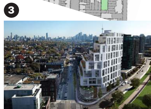
3 1181 Queen Street West 15 ST Under Construction
