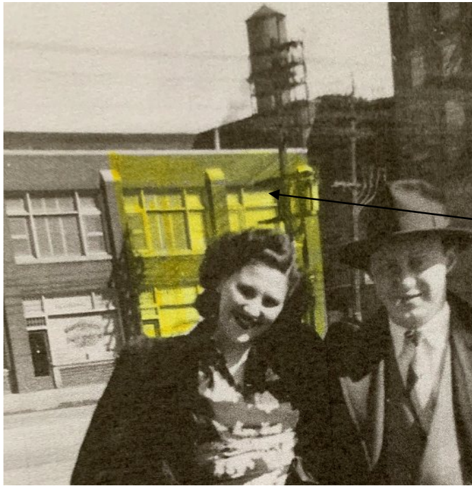
17. Photo of building south end prior to the removal of the south 2 bays. 147 Spadina was initially constructed symmetrically around the front entrance
