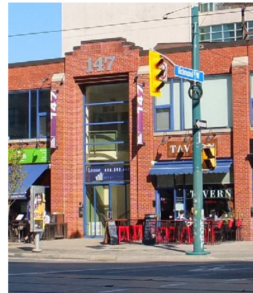
23. The same view today. Note the loss of the Art Moderne entrance surround and the historic window patterns. This diminishes the design significance of the building. PGA
